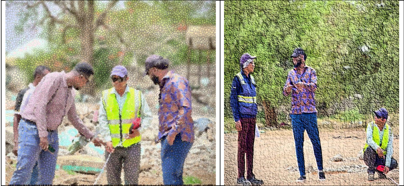
Figure 5 During the screening assessment of Hirshabelle State CSC office construction site
